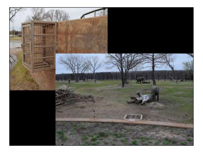
Hay feeders are mounted to the walls. They require the elephants to eat at the walls, near the public. They are also easily accessible to the keepers.
